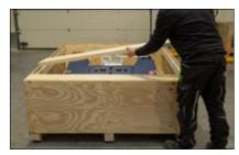
Remove the remaining bolts from the front cover and take it off.
