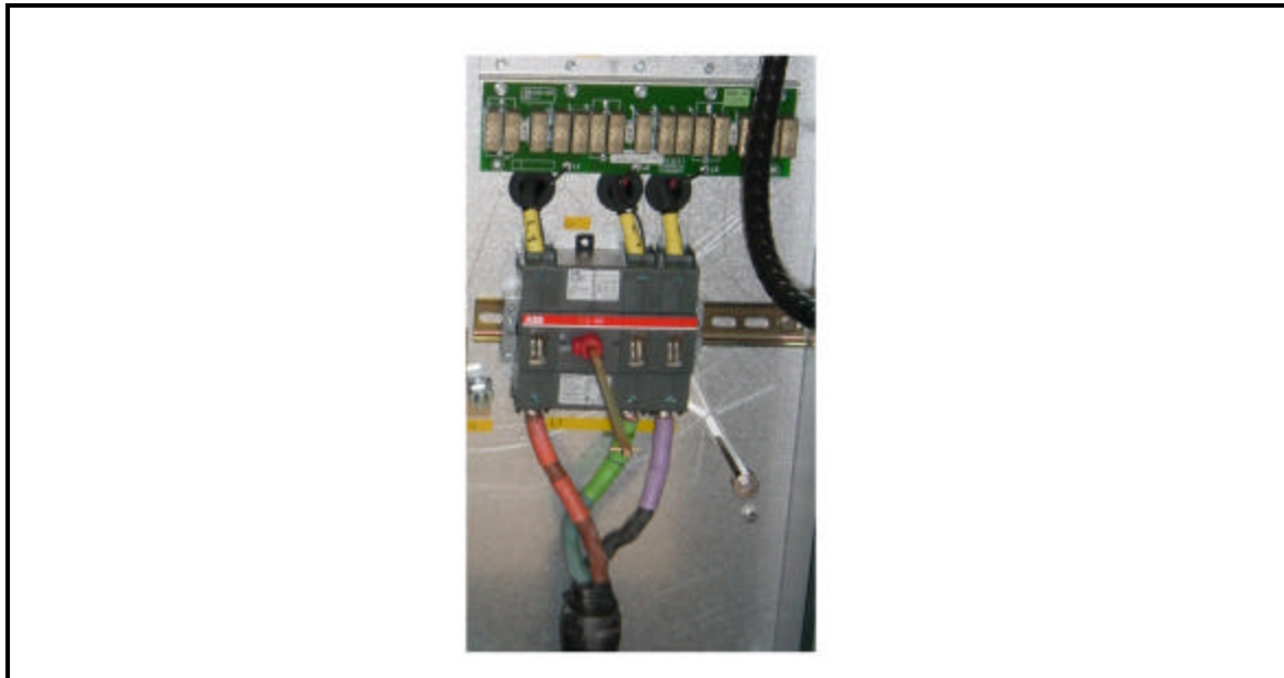
Input Cable Connections Figure 2
